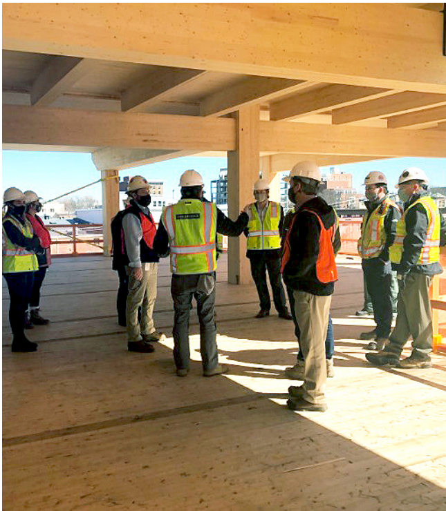
Figure 2. Apex Building under construction. Virginia Dept. of Forestry
